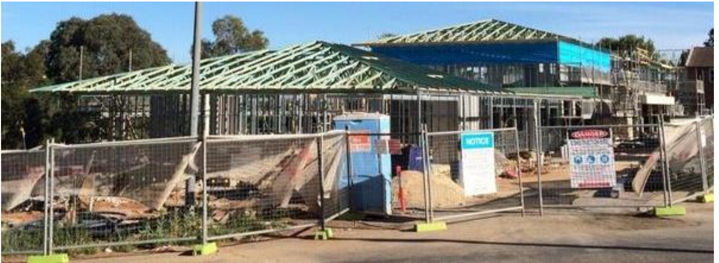
Ground floor roof trusses go up ready for the roof
