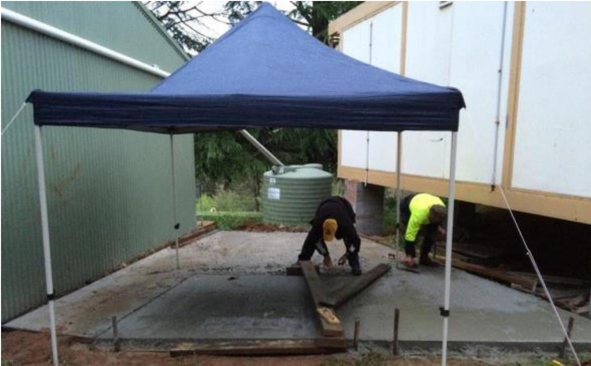
Making good use of the tailings from the big concrete pour at #YHSRebuild, Mr Hansson and Paul finish the shed slab.
