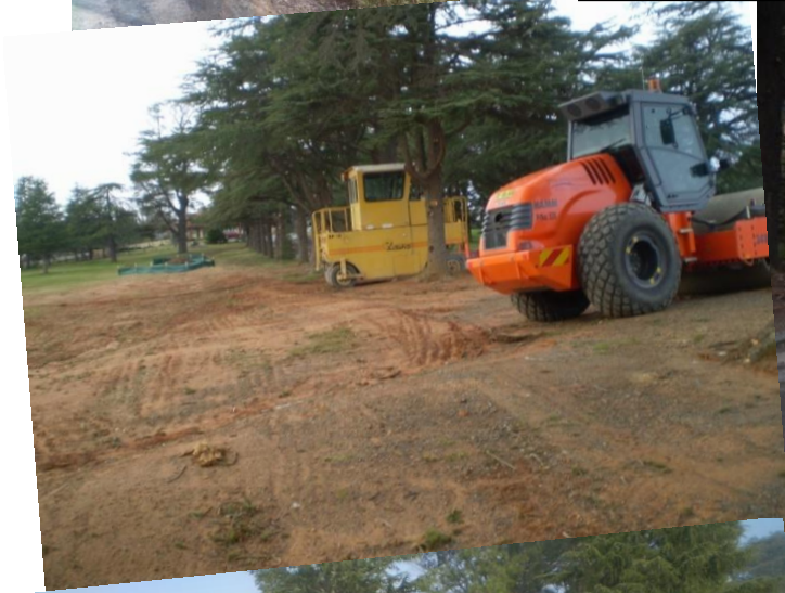
Roadwork at Yass High School
