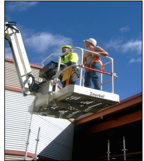
Casey Edwards tying the elevated platform
