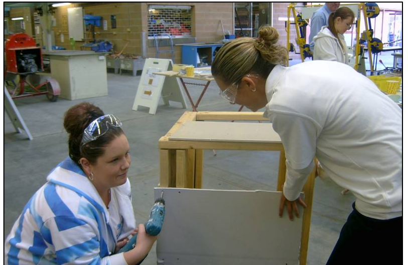
Megan Cooke assisted by Peta Stokeld to attach a plaster sheet to a frame in the Plastering workshop
